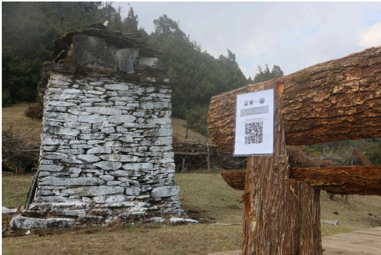
QR code installed near the Lhasey Kuntu Lekpa stupa along Mindrula to Jigmeling trail.
